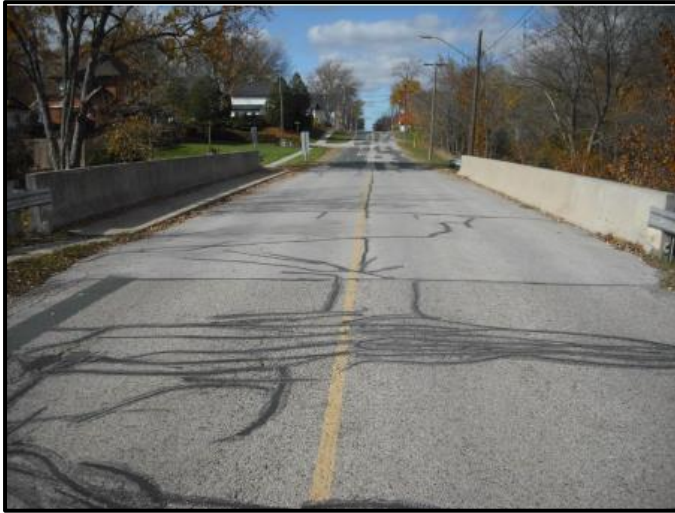
Main Street Bridge (BCI = 98.8 Very Good)
