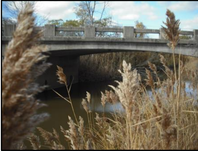
18/19 Side Road Bridge (BCI = 86.6 Very Good)
