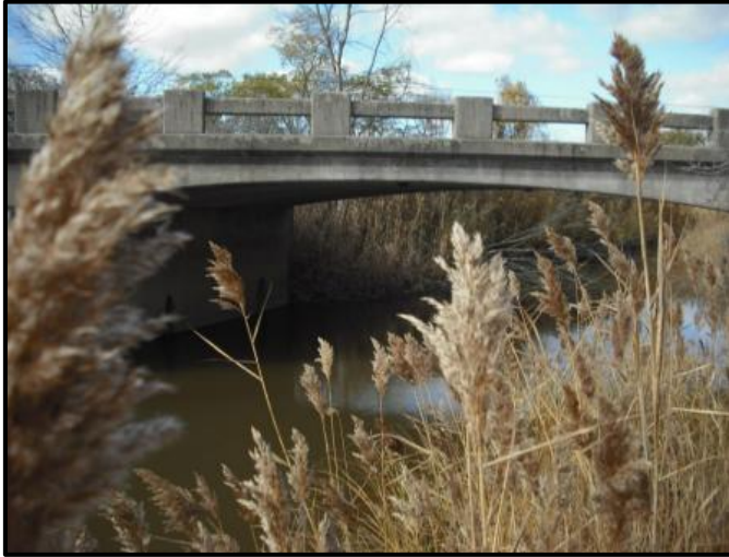
18/19 Side Road Bridge (BCI = 86.6 Very Good)
